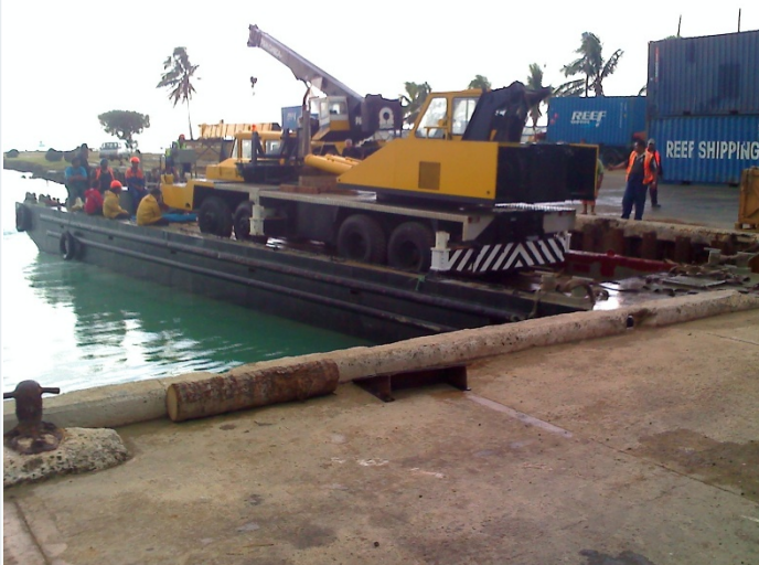
The new crane delivered by the Southern Express to Aitutaki
